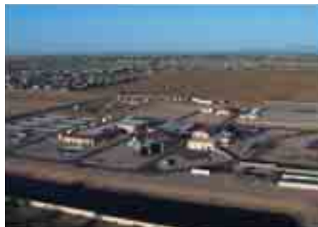
Santan Vista Water Treatment Plant
